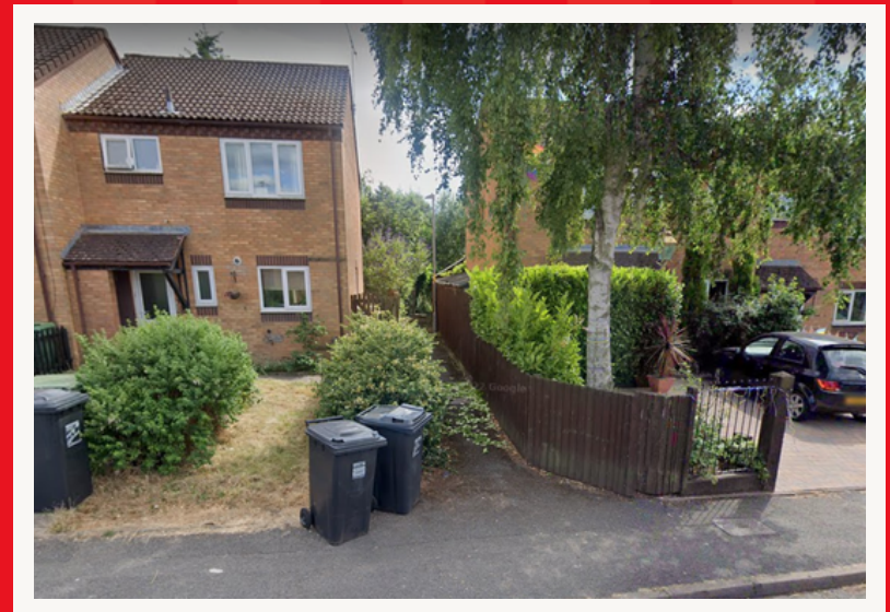
Entrance to Cedar Road turnstiles
